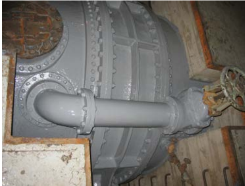
→ Penstock coated with anti-corrosion coating Belzona 58II
