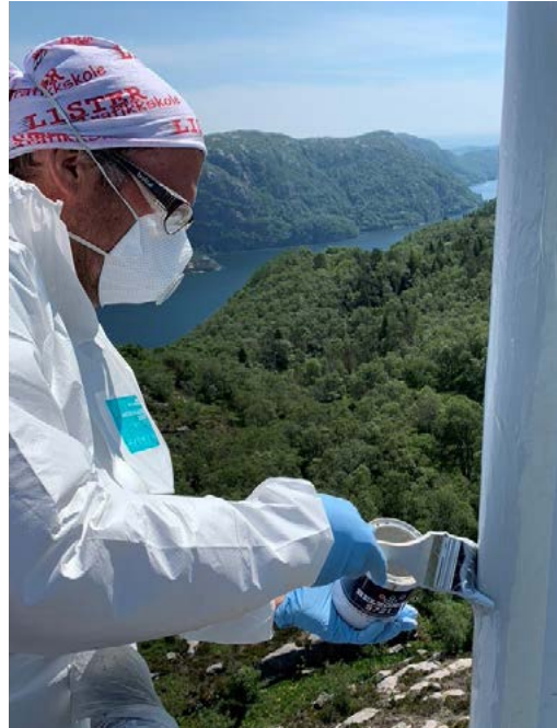
← Belzona 572I provides leading edge protection on a wind turbine blade
